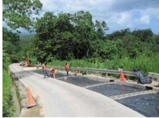
Klehm's Hill – just below the corner halfway up the hill – preparing the pavement panels for pouring. This work is now 75 % complete.
